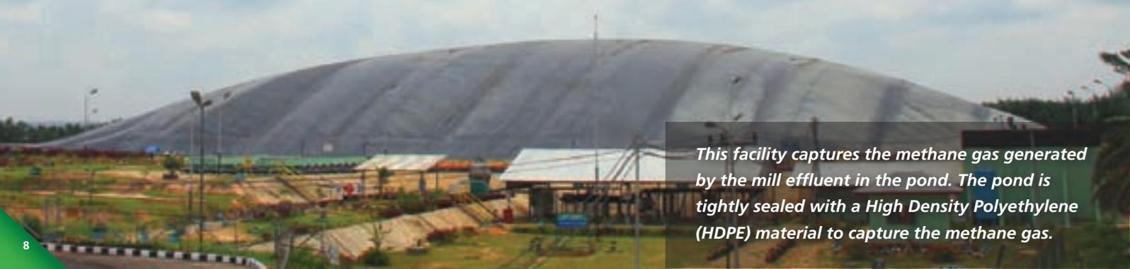
*This facility captures the methane gas generated by the mill effluent in the pond. The pond is tightly sealed with a High Density Polyethylene (HDPE) material to capture the methane gas.*
